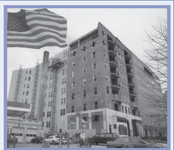
Construction underway to double Heritage's size on Capitol Hill.
